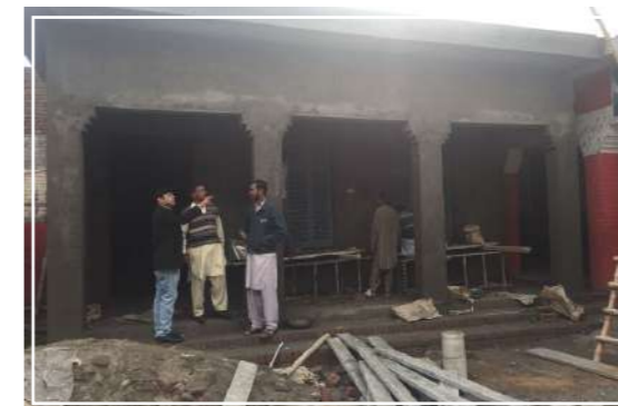
Construction of the project
