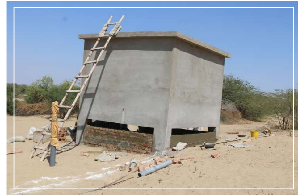
Construction of the project
