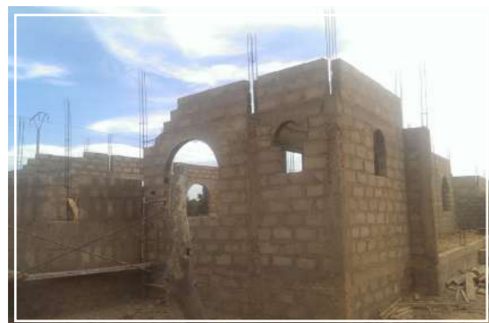
Construction of the project
