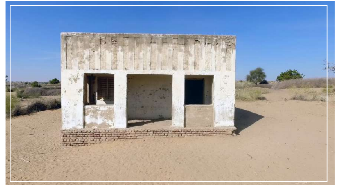
One classroom school
