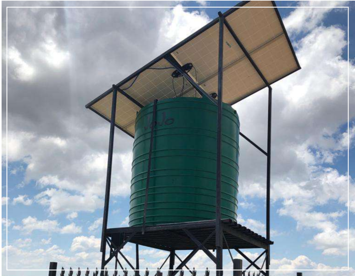
Solar Panel Water & Power Centre
